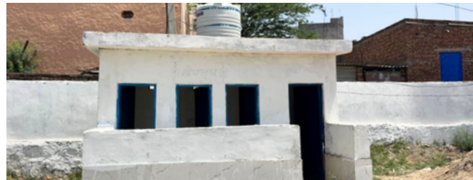
Sanitation Unit Construction with water facility
